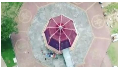
Pagoda Roof (Problem 1)
